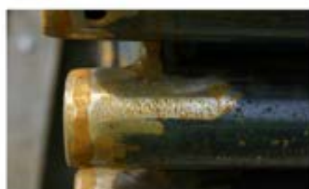
Weld ground flush
