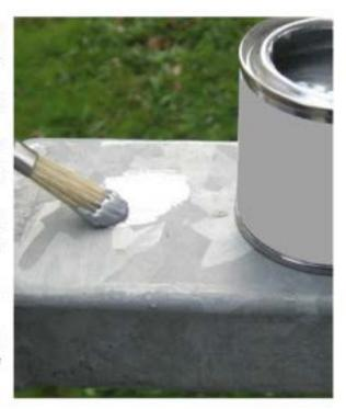
In practice, most repairs are conducted using a zinc-rich paint which might be brush or aerosol applied. It is also common to use a sprayed final top coat to attain a more aesthetic finish. Ideally the product used should contain at least 80% zinc by weight, the key being to follow the manufacturer's instructions and ensure sufficient coatings are applied to achieve the 100 µm repair coating thickness requirement of BS EN ISO 1461: 2022.
