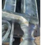
Note: When cast iron is welded to mild steel there needs to be sufficient weld as differing material composition can lead to cracking of the weld.
